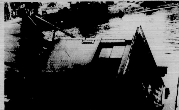
Watered down — This view of the collapsed Belleville bridge boathouse shows the weakened structural steel supports which may have precipitated the incident. (Photo by Christopher Ruffini)
